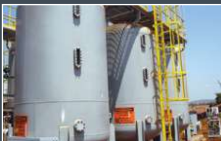
Ion-Exchange Demineralization System Moa Nickel, Cuba
