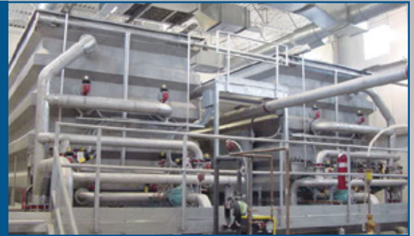
Gravity Filter Trains Limoges Canada
