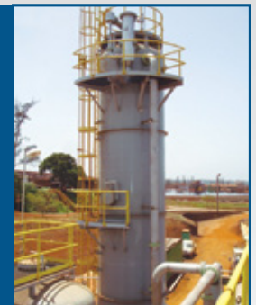
Vacuum Degasifier Moa Nickel Cuba
