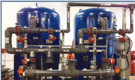
Pressure Filtration System Rocky Rapids Canada
