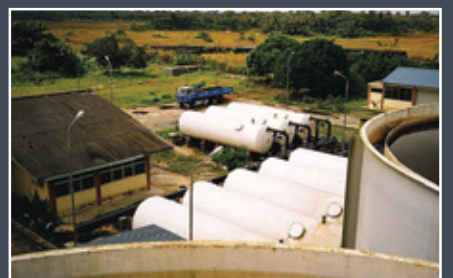
Horizontal Pressure Filters Lagos, Nigeria
