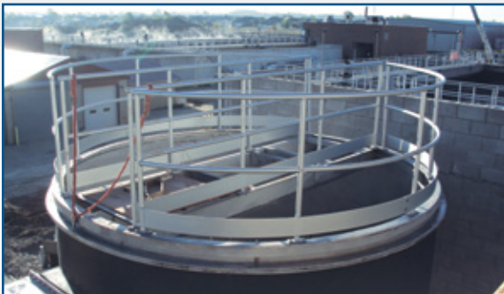
Vortex Grit Removal System Belle River Canada
