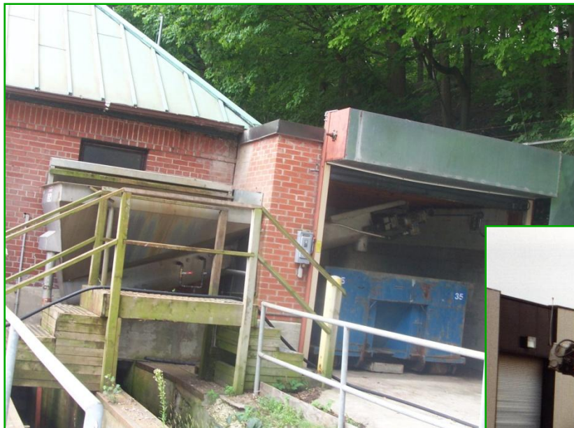
▲ North Toronto WWTP, Ontario, Canada
