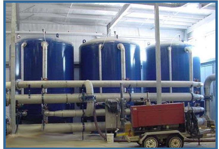
▲ NR-GAC Tower – South Chatam Ontario, Canada Design Flow of each tower: 7600m 3 per day
